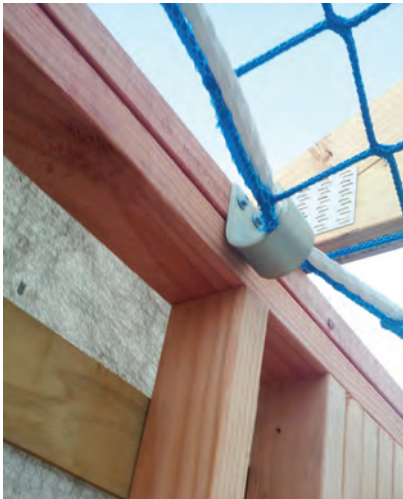
Fasten Hooks with 2 x M8 x 1.25 x 40mm Fasteners for Timber Framing.
